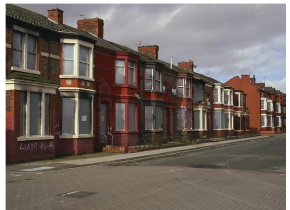
A street of boarded-up houses awaiting demolition, an increasingly common sight throughout Merseyside
